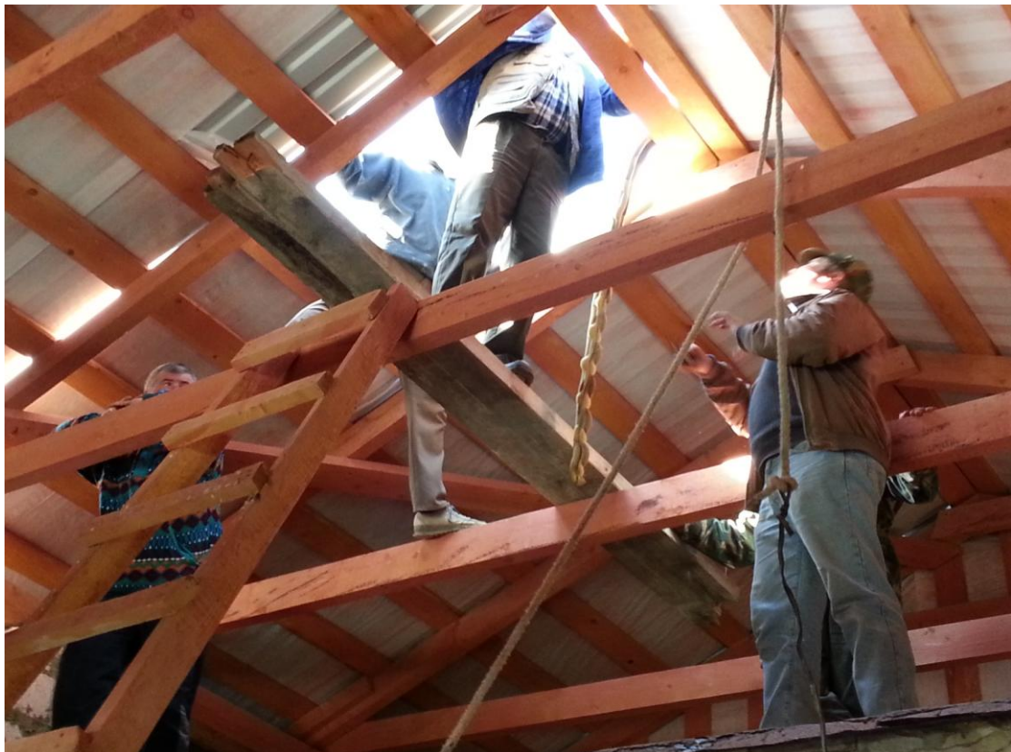
The siren mast was installed on the attic and was led through the roof.
